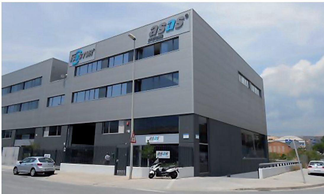
Edificio de ASAS Systems en Sant Boi, Barcelona. ASAS Systems offices in Barcelona, Spain.
